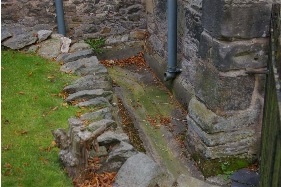
Figure 5: West wall of porch prior to excavation
