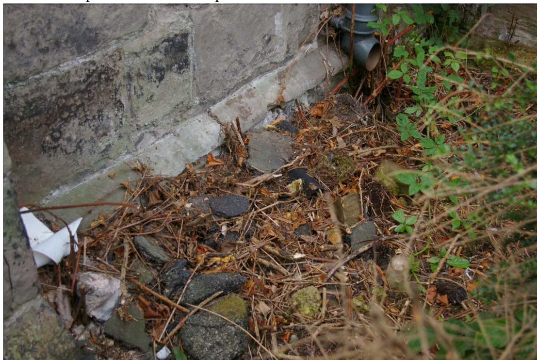
Figure 7: East wall of porch prior to excavation
